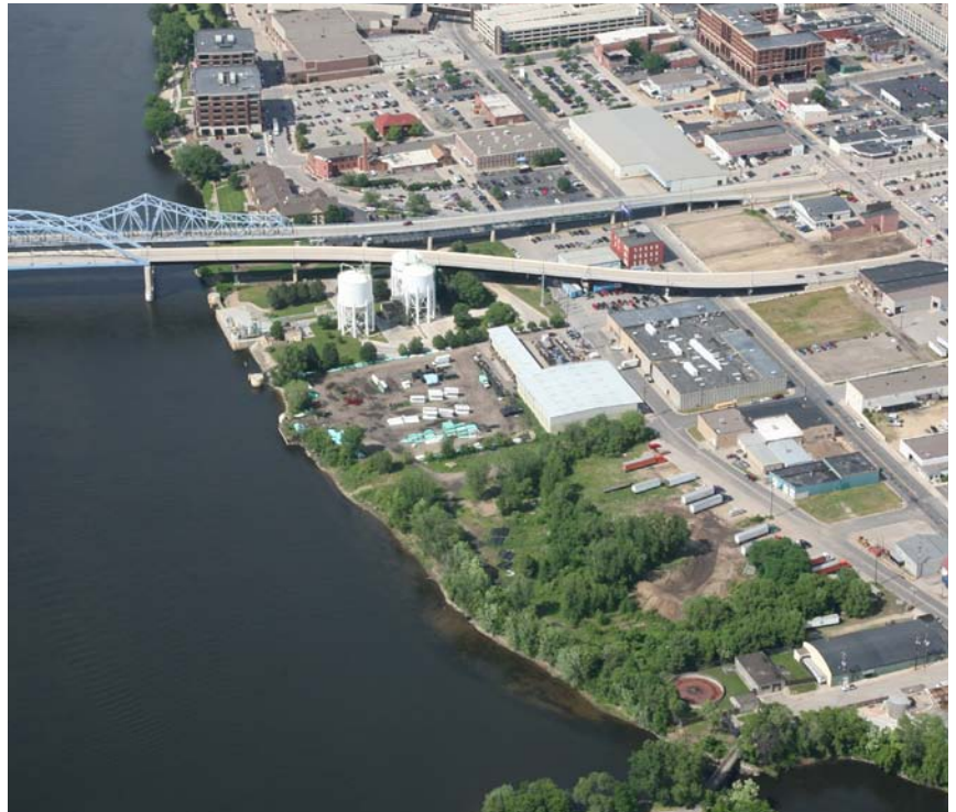
First Supply Plumbing (Division Street Dock)
