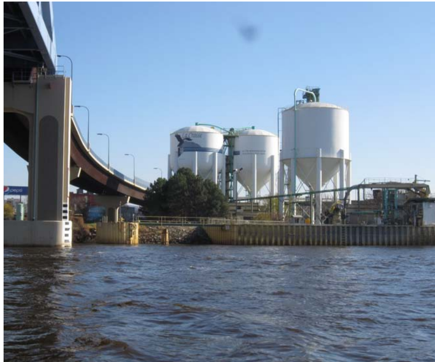
Division Street Dock from water
