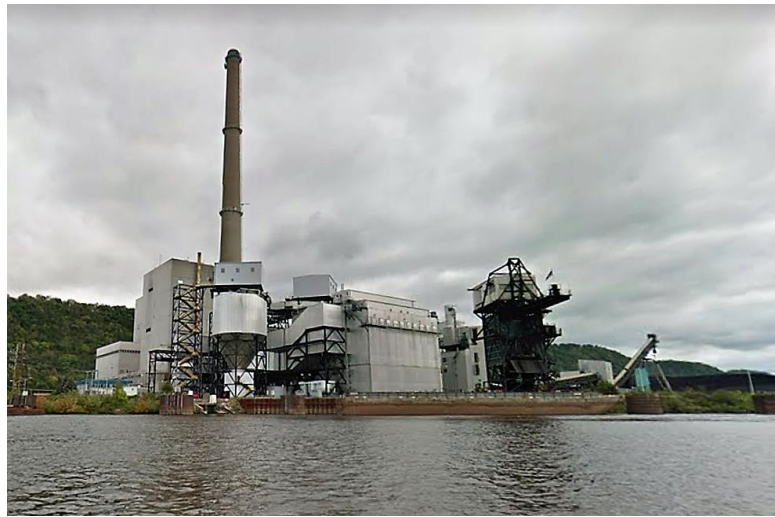
FIGURE 24 DAIRYLAND POWER PLANT – GENOA, WI
