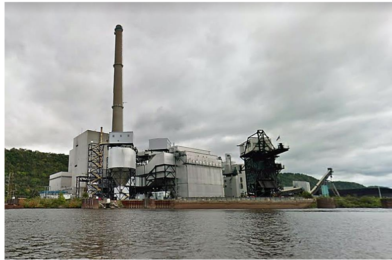
FIGURE 24 DAIRYLAND POWER PLANT – GENOA, WI
